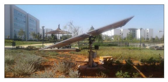
1,2 kW Pilot project off-grid solarwater pumping irrigation systems - Rabat - Morocco
